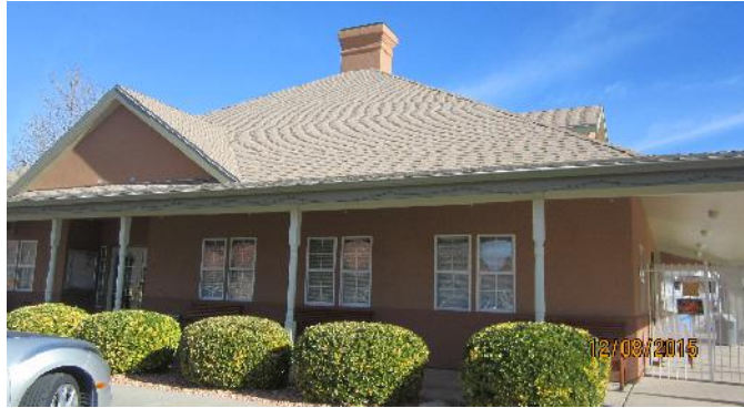
The roof was replaced in 2014. The useful life is approximately 25 years.
