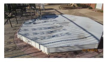
Spa - Deck Caulking, Deco-Seal, Repl. We have budgeted for this every 12 years beginning in 2024. Expansion joints should be replaced at this point.
